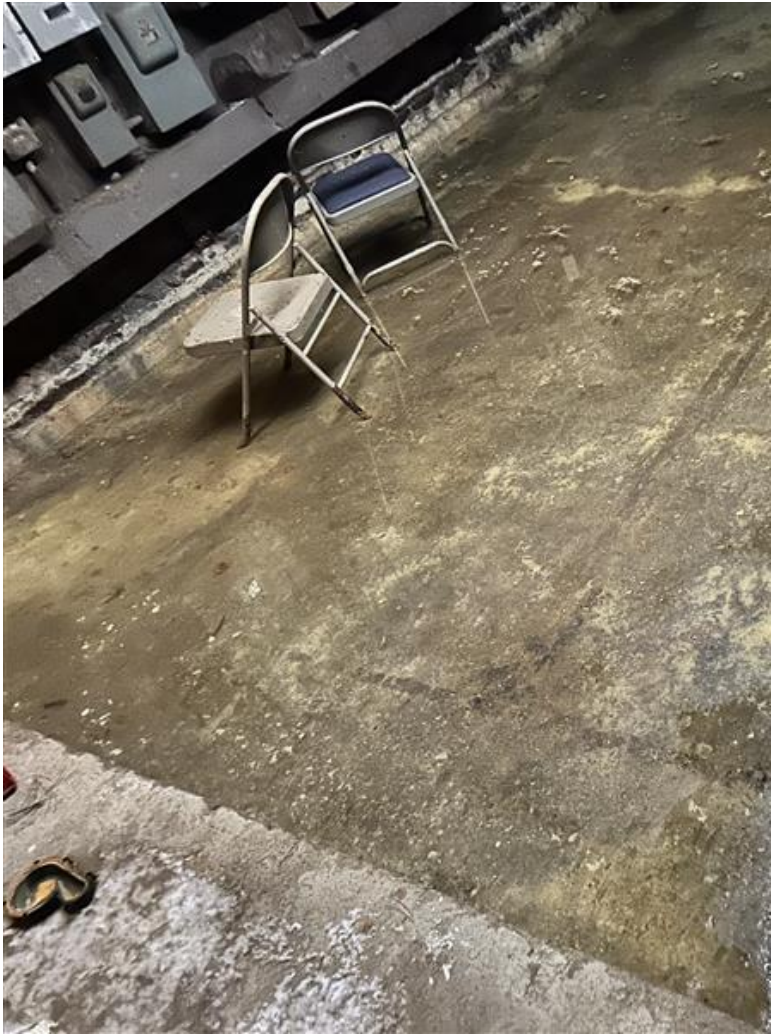
3-4" OF STANDING WATER IN BASEMENT UNKNOWN SOURCE
