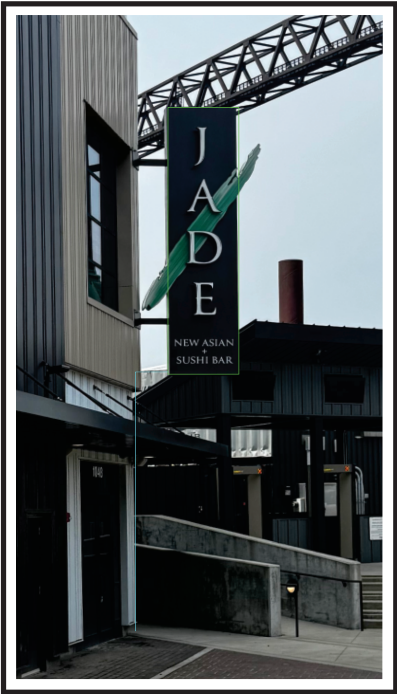
EXISTING ELEVATION SCALE 3/16" = 1'-0" RE-USE EXISTING ARMATURE (2) 12" X 24"- 1/2" 90 DEGREE ANGLE STEEL PLATES WITH 4" X 4" TUBE BRACKETS 20" EXTENSION TO SIGN 9'-0" ON CENTERS
